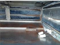
2nd STEP: remove the dirt from the tray with jet wash.
