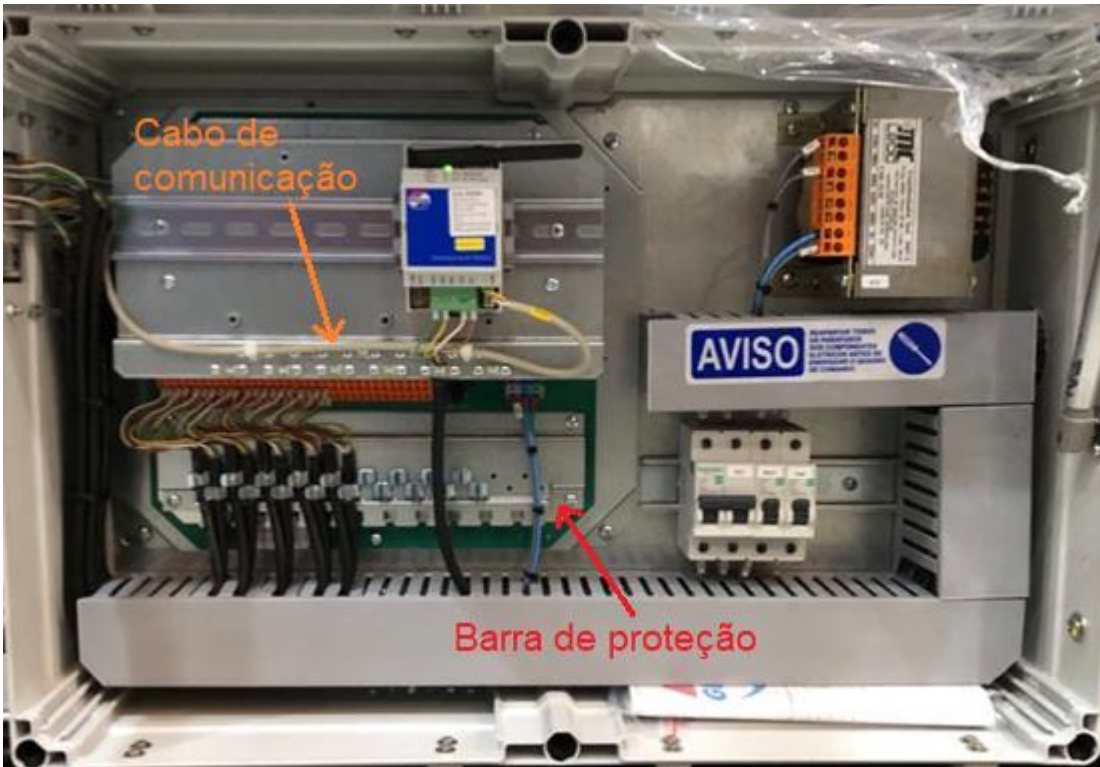
Figure 2: Internal panel without GMM display.
